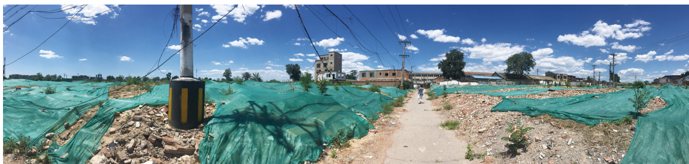
Photo 4. In the aftermath of the demolition of a peri-urban village between Beijing's fourth and fifth ring roads, June 2019. Credit: Photograph taken by the author.
