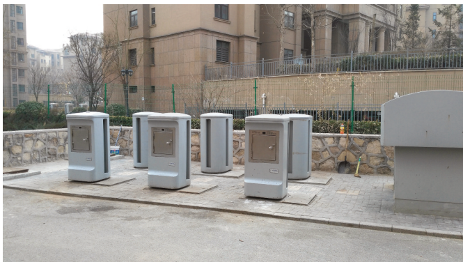
Photo 1 – Pneumatic rubbish collection points in a residential quarter of the Tianjin eco-city.
